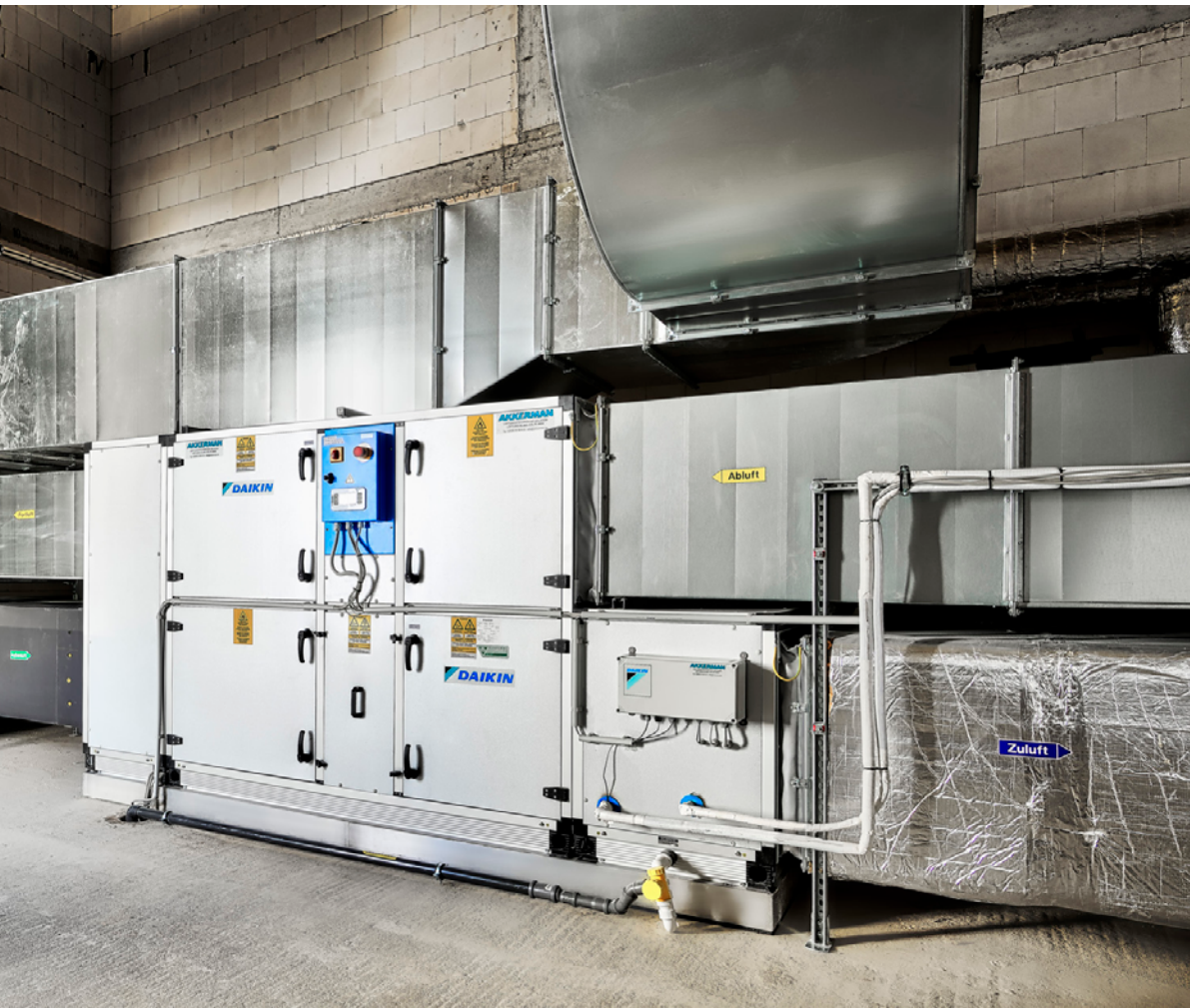
D-AHU Modular R installation
