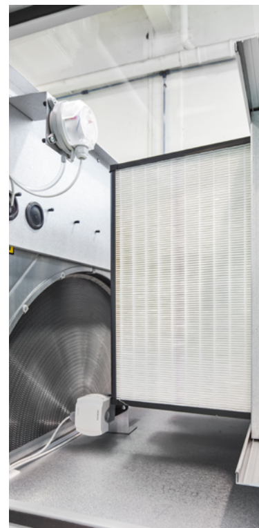
Heat recovery wheel and filter
